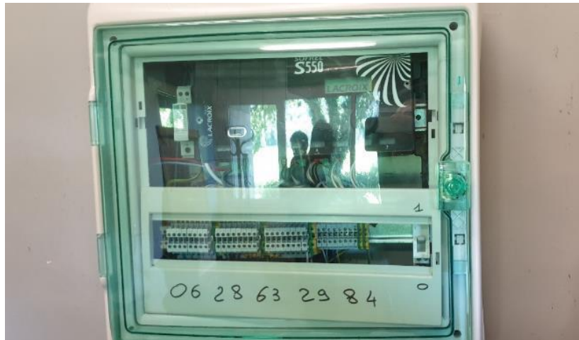
Figure 21 – Boîtier de communication SOFREL (RTC & GSM)
